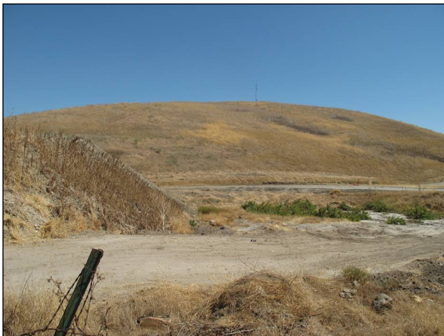
Figure 4. Soil deposition to the left and constructed road in the background at EO 1.
